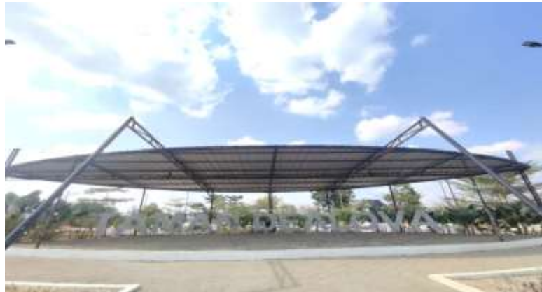
Figure 2 Front View of Dealova Park, Pangkalpinang City
