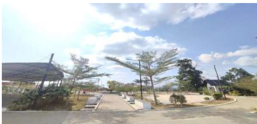
Figure 5. Condition of Seating Facilities at Dealova Park, Pangkalpinang City
